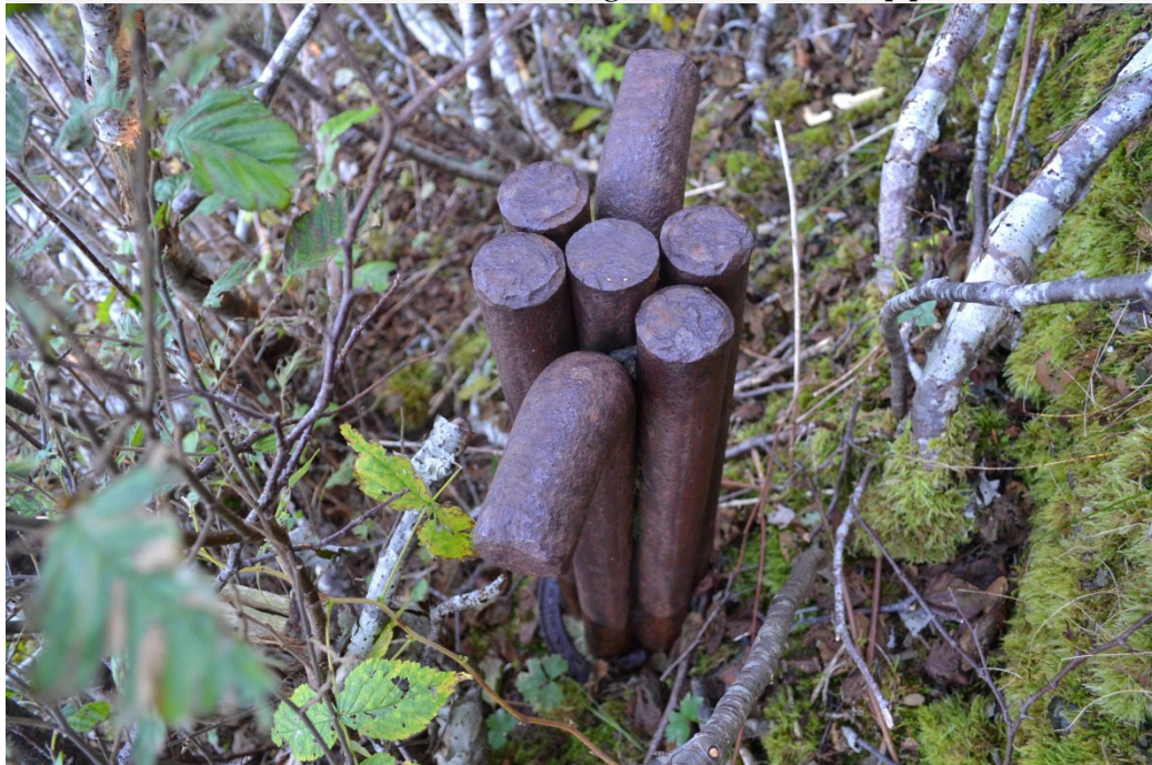
Figure 7: A possible anchoring or mooring fixture made from 7 metal rods held together inside a buried pipe.
