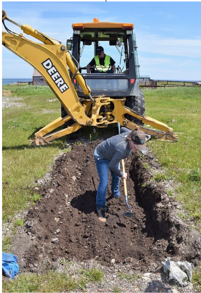
Figure 2: Field director, Catherine Losier, unearthing the 2017 excavation.
